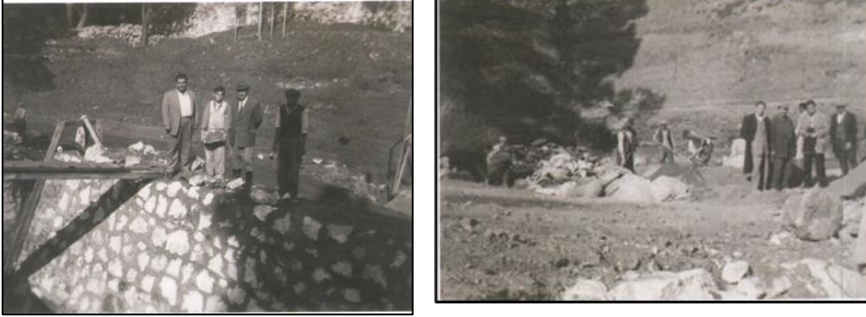
Figure 9. The water tank construction works in the Bursa Mevlevîhâne garden, 1953 (Elbas & Alkan, 2023, 37)
