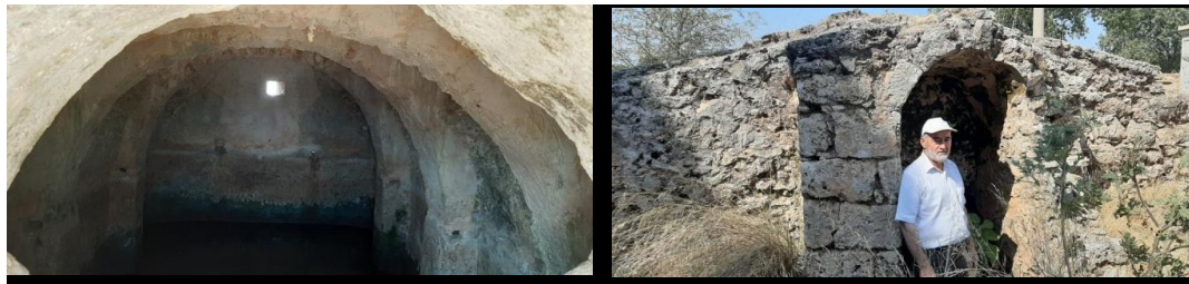
Figure 14. Çıplaklı Neighbourhood Cistern and Cistern Interior (Original Photo: Öncü, 21/03/2022).
