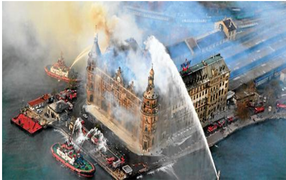
Figure 1. Haydarpaşa Train Station burned down on 28 November 2010 due to a short circuit in the electrical installation (Source: www.denizhaber.net )
