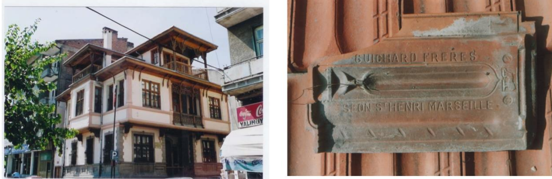
Figure 1. Marseille type tile on the east facade and roof of Notary Ragıp Anadolu Residence (Aygör, 2015)
