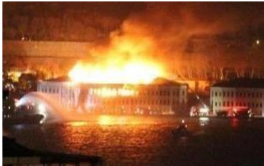
Figure 3. Galatasaray University burned down on 22 January 2013 due to a short circuit in the electrical installation (Source: www.yesilgazete.org )
