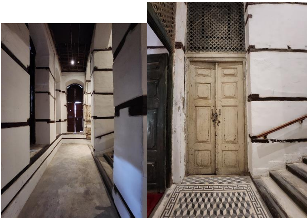
Figure 9: Conservation and restoration process of floors, doors, and windows, (by Author)
