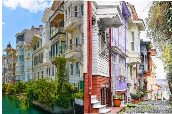
Figure 4- 5. Historical buildings of Arnavutköy neighborhood (Tekkol, 2021)
