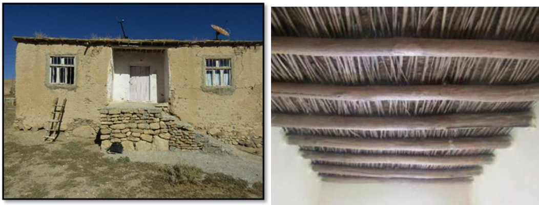
Figure 20. Wood is used in ceiling tiles, door and window openings
