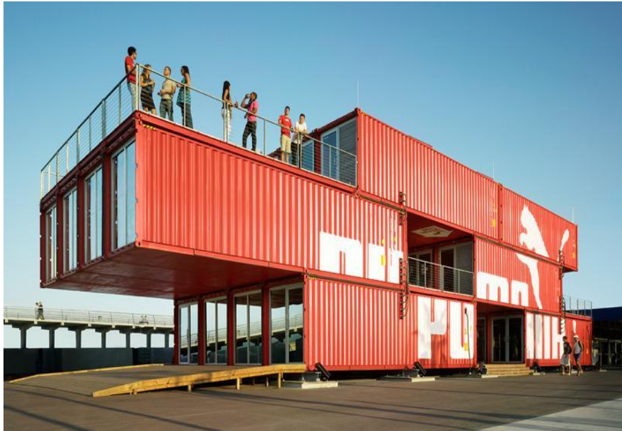
Figure 4. Transformation of disaster containers into youth centre (Keskin, 2015).
