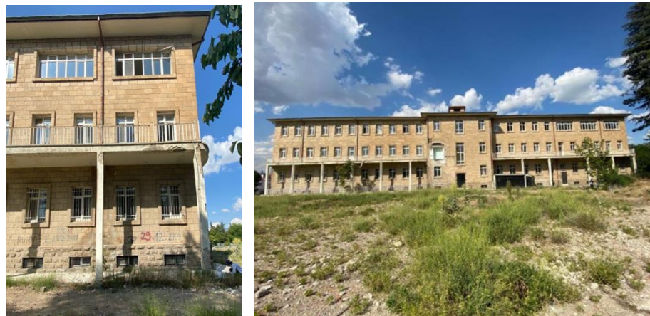
Figure 3. Rear view of the rectorate building
