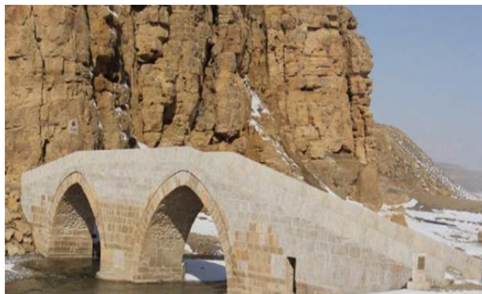
Figure 3: Kelegom Bridge (URL-3)
