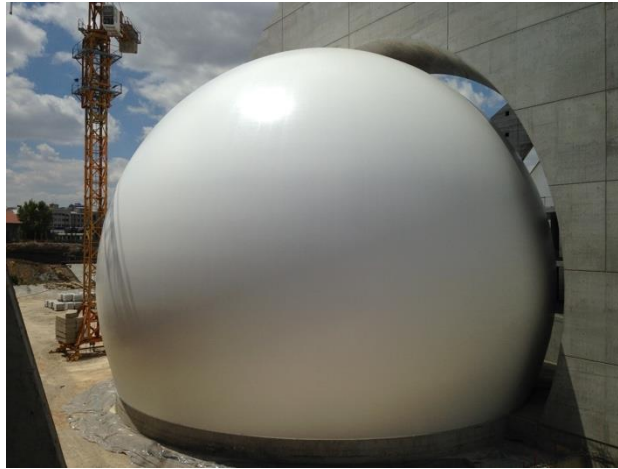
Figure 10. Construction site photograph. pneumatic formwork. (Uygur Architecture Archive)
