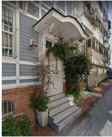
Figure 10. A building entrance in Teyyareci Suphi Street (Google Maps)
