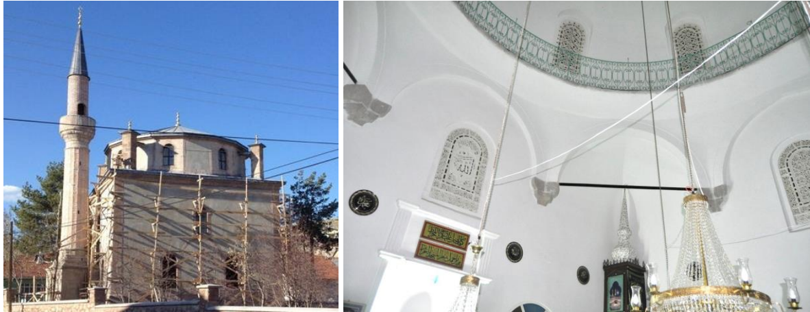
Figure 3. Exterior and interior view of Hatipler Mosque (Karakuş, 2012)
