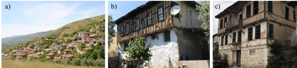
Figure 1. a) General view of Ömerli village, b and c) examples of traditional Turkish houses in the village; mud-brick-filled straw structures (Bozyel, 2019)
