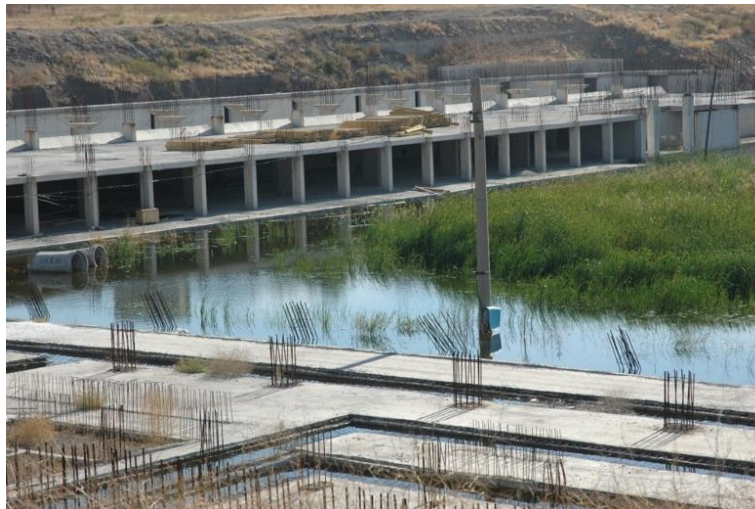
Figure 11. Groundwater resurfacing during the pause period (Uygun Architecture Archive)
