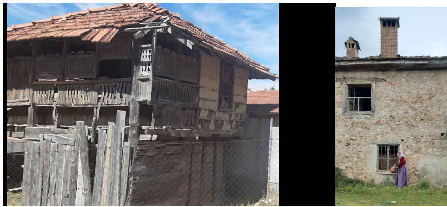
Figure 16. a. Dağbeli Neighbourhood Traditional Architecture, b. Kömürcüler Neighbourhood Traditional Architecture (Original Photo: Öncü, 2022).
