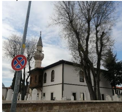
Figure 13. Mosque southeast facade (Demirkol, Burçin İrem Demirkol Photo Archive, 2023)
