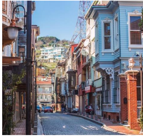
Figure 8. Historical buildings of Arnavutköy
