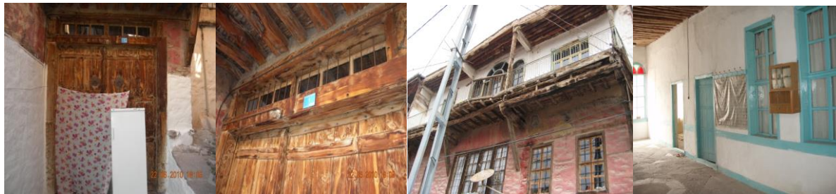
Figure 15. The ground floor features a double-winged wooden sentence door of the building, wooden handrails supporting the protrusion on the south facade, and the upper floor's inner living area with rooms (Sille Street Rehabilitation Survey Report, 2014).
