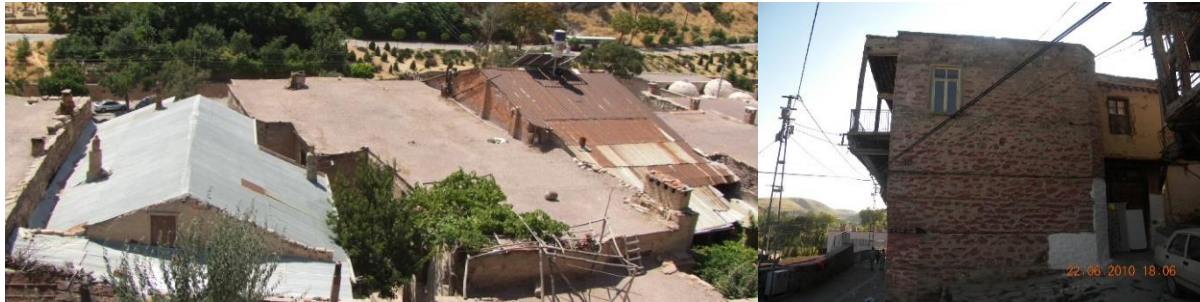
Figure 16. The contiguous layout and orientation of Hacı Ali Ağa Mansion towards the south and east facades (Sille Street Rehabilitation Survey Report, 2014).
