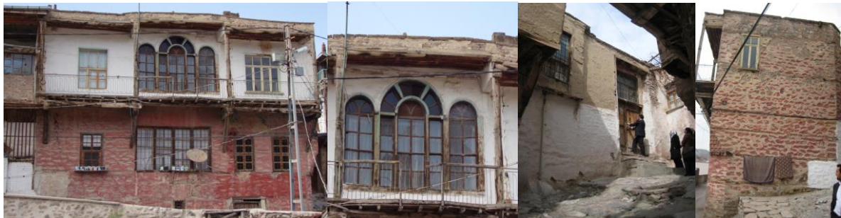
Figure 20. The Protrusion With Round-Arched Windows on the South Facade and the Eastern Facade of Hacı Ali Mansion (Sille Street Rehabilitation Survey Report, 2014)
